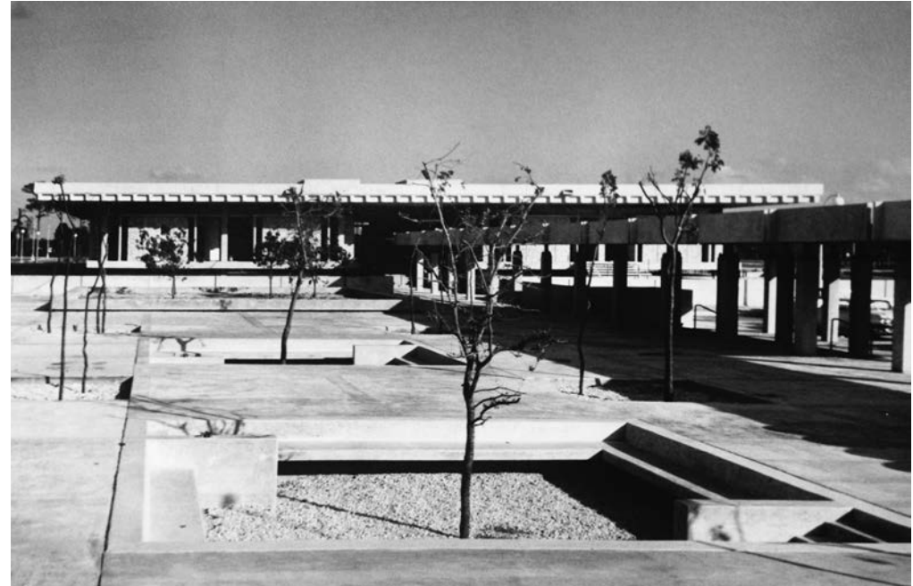
Miami Dade South Campus / Photo: Miami History Museum / Architects: Pancoast, Ferendino, Grafton, later Spillis and Candela
