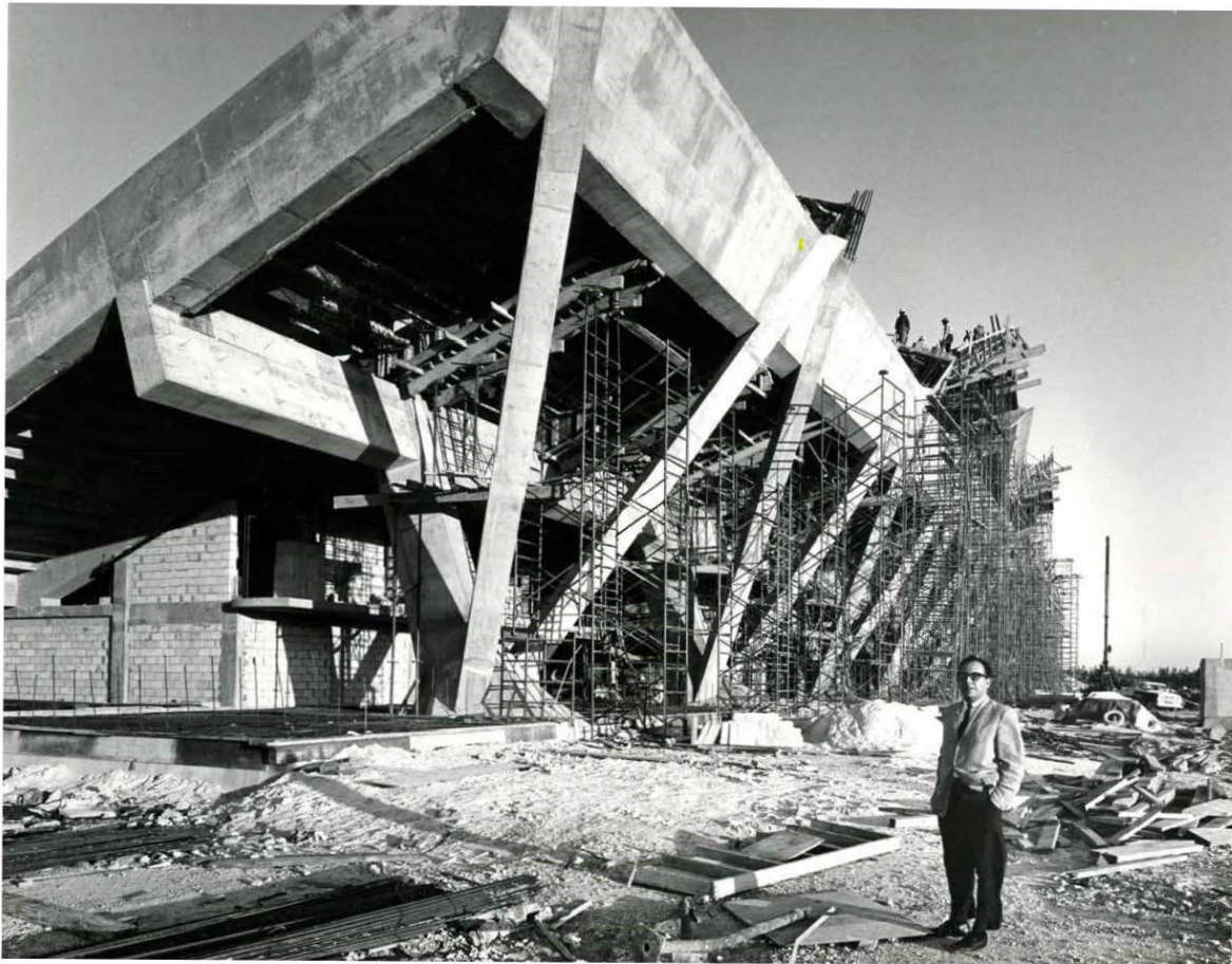
Miami Marine Stadium under construction with 26-year-old Architect, Hilario Candela
